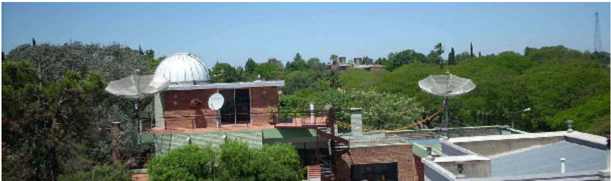
Figure 1 A general view of the northern facade of the observatory after embracing the radio experience.
